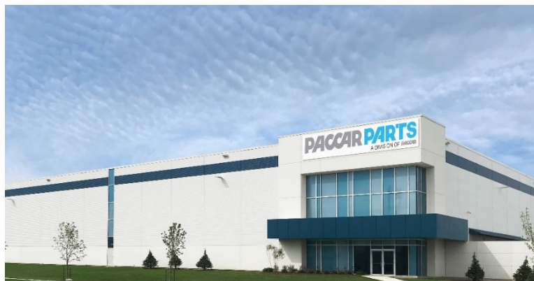
PACCAR Parts Distribution Center in Toronto, Canada
